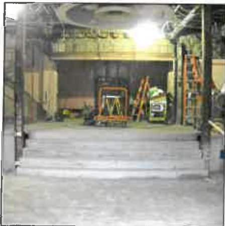
In - Progress Lobby
