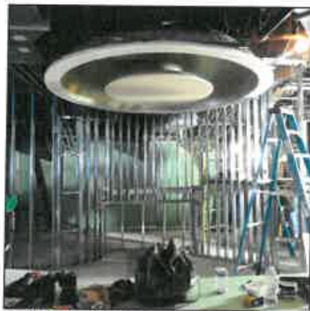
In - Progress Bar Area
